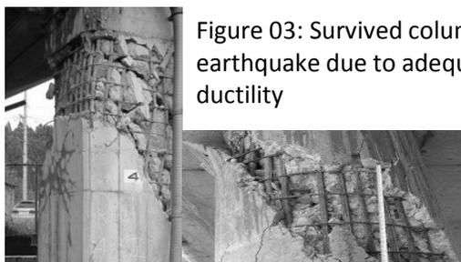
Figure 03: Survived columns after earthquake due to adequate ductility
